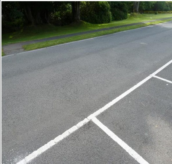
IMAGE 5 – Deterioration in Wheel Track
